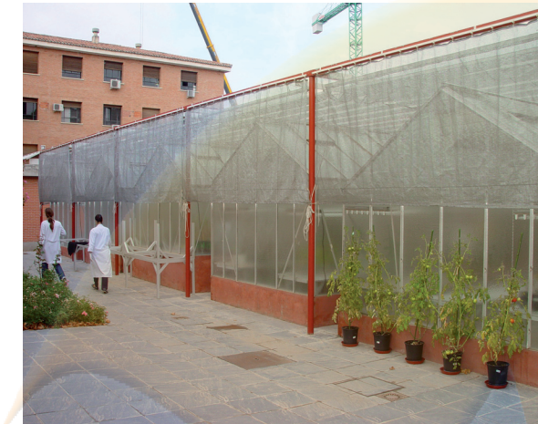
Greenhouses and Growth Chambers
