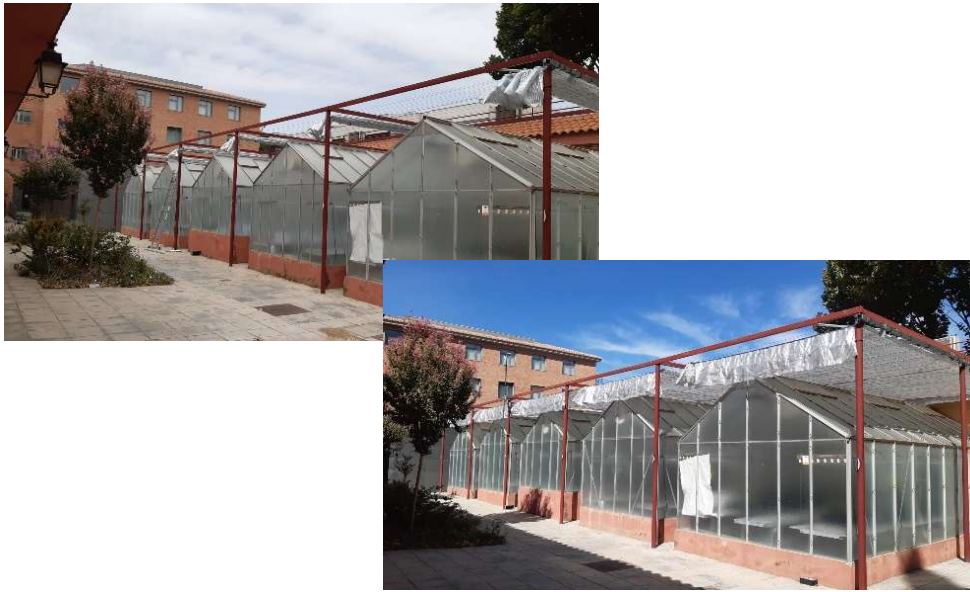
New automated greenhouse cover awnings
