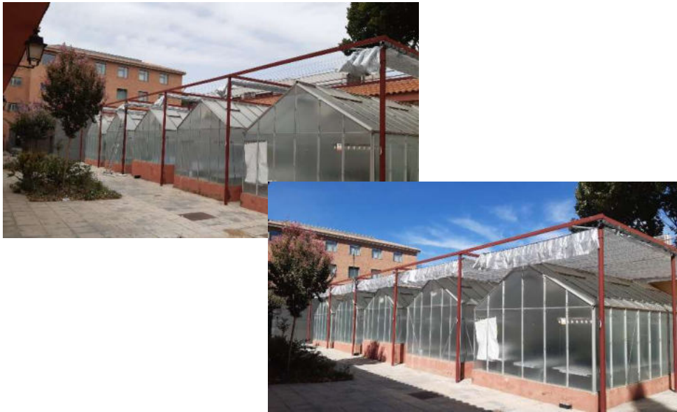
New automated greenhouse cover awnings
